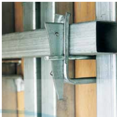
Wedge type form tai and backing plate K-II
